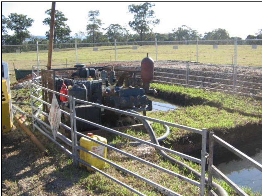
Plate 2: Reticulation Pit Showing Pumping System, safety fencing and man-proof fencing.
