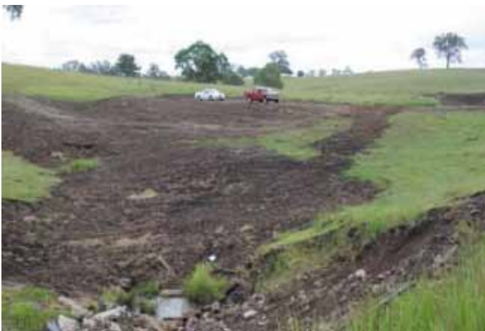
Downstream of dam wall showing the bypass trickle pipe outlet.
