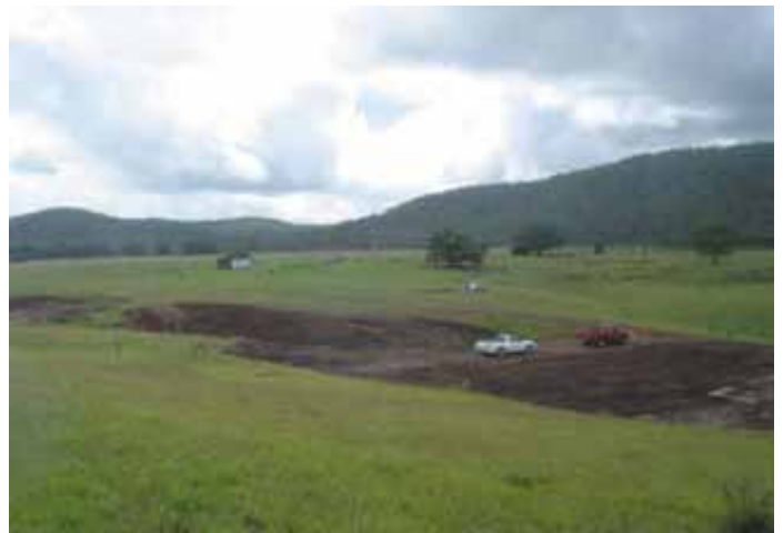
Looking down onto the dam walls shortly after completion.
