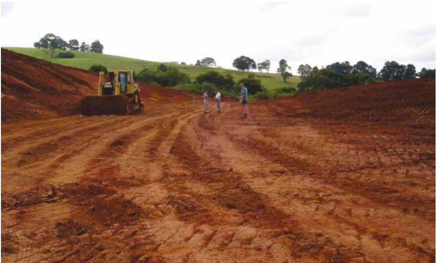
Checking the spillway width to ensure flood flows can be released.
