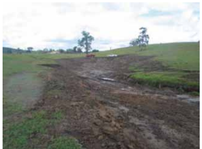
Dam wall looking downstream. Internal excavation increases stored volume.
