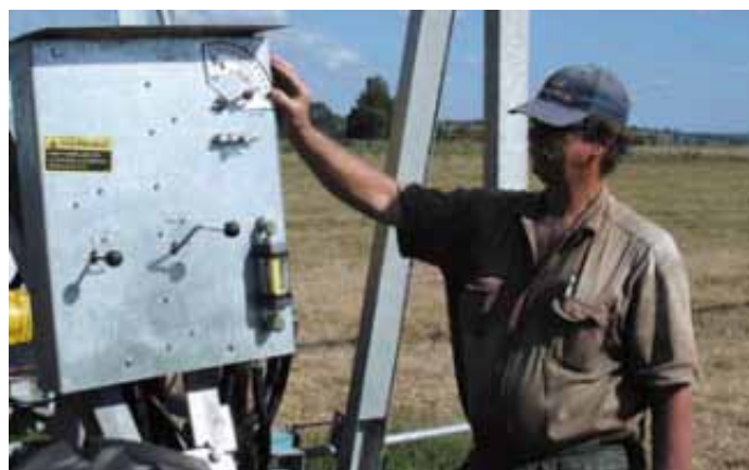
The control panel which allows Ric to set different irrigation rates as well as control direction of travel.
