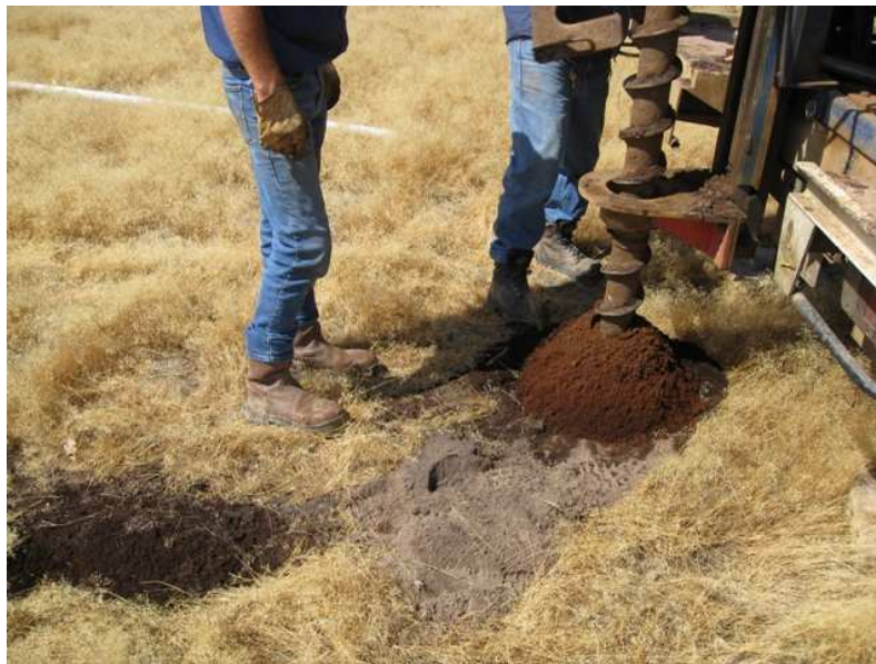
Drilling at Gngangara Mound
