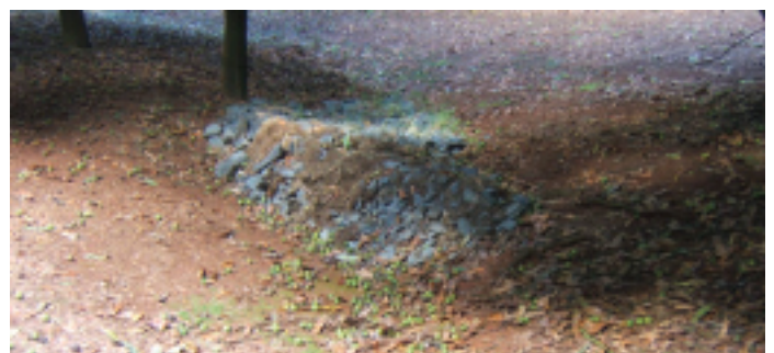
A small check dam protects where water crosses the tree line
