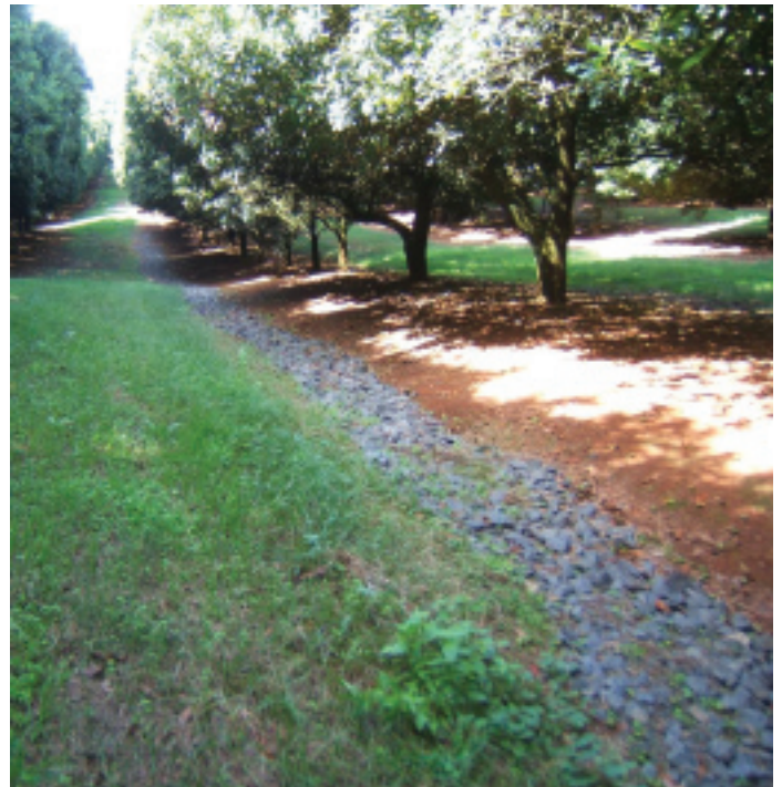
Rock fill in a gully protects against further erosion
