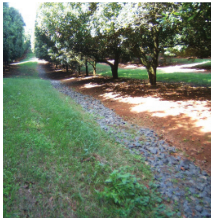
Rock fill in a gully protects against further erosion
