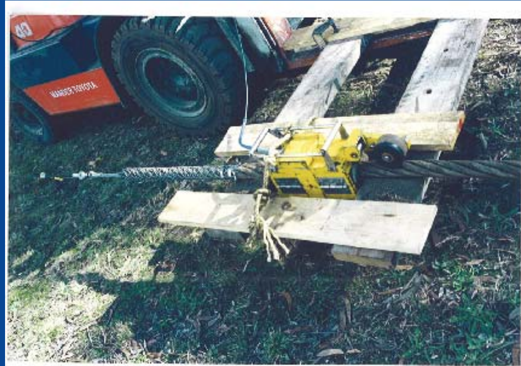
Photograph No. D26 – NDT set-up
