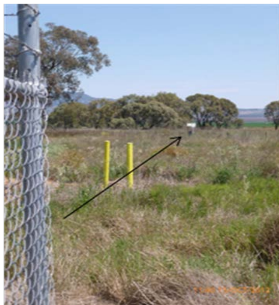
Figure 3: Signage of pipeline through the property 'The Point'. Grazing is permissible over the pipeline (arrow indicating pipeline direction).
