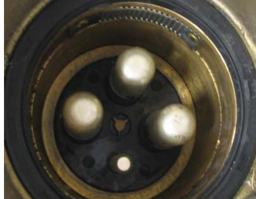
Photo 2. 425A pins and 425A orientation
