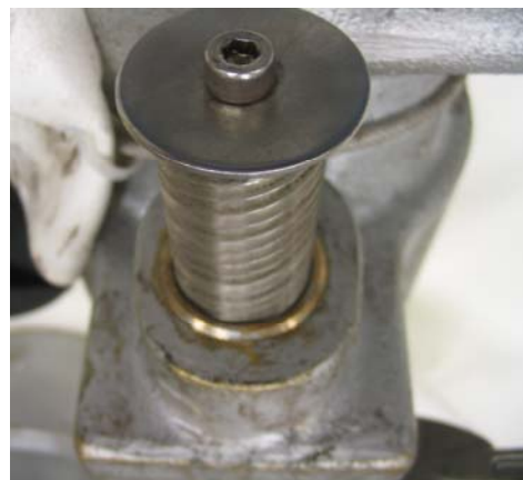
Photo 4. Jacking screw in a case with a bushing - UNACCEPTABLE ARRANGEMENT
