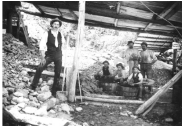
Washing pieces of ore by hand, Pampula, c1890
