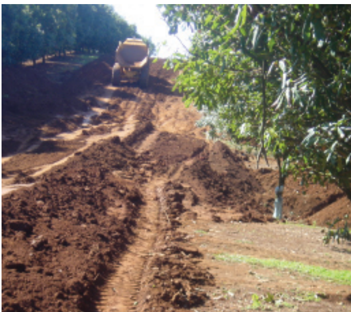
The diversion drain is formed
