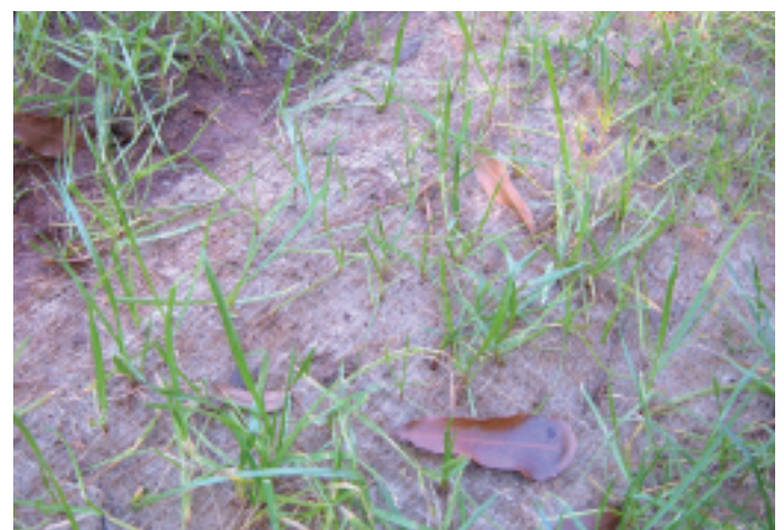
Grass growing through the erosion matting
