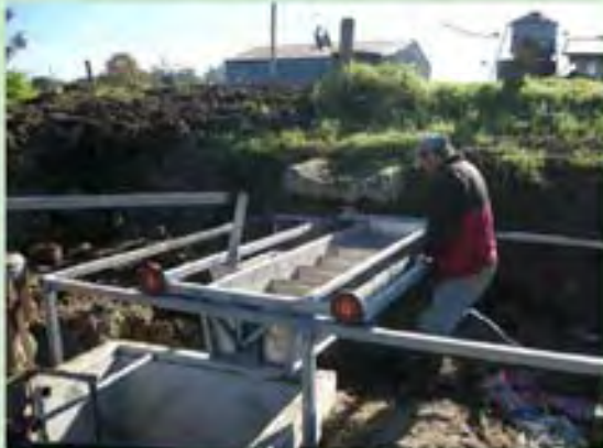
Above: (Lee & Clarke family) Stone- trap being installed
