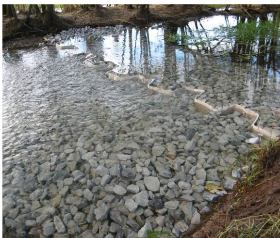
Vinyl sheet piling was used for the weirs (as seen in ASSAY #50)
