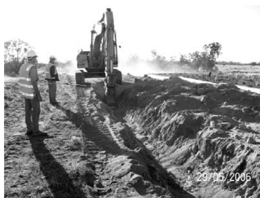
Construction on the pipeline. Employees of Mitchell Australasia at work.
