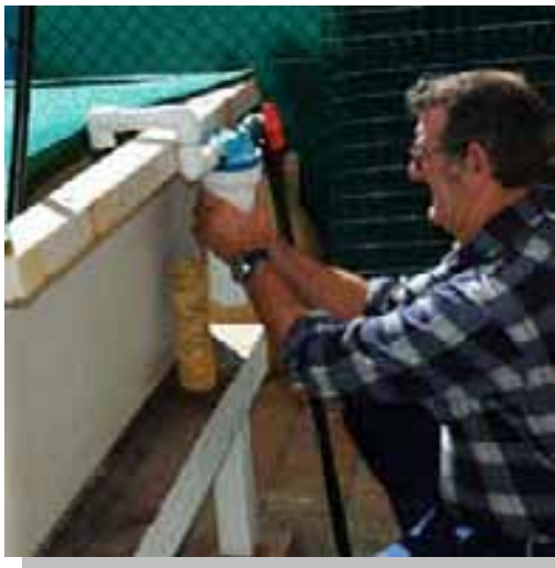
Figure 35 Nursery tank filter element being changed.
