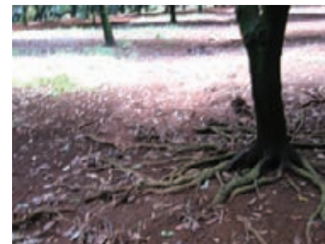
Exposed tree roots
