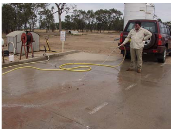
Wash excess mud from the wash down pad
