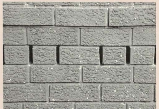
Figure 5. Spaced brick ventilation.
