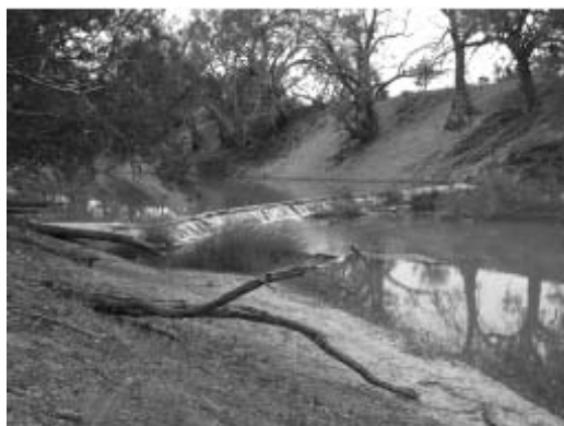
Below: A two cell vertical slot fishway
