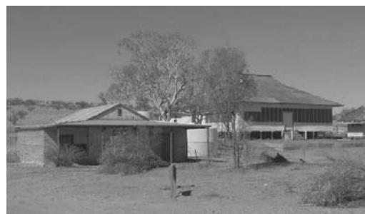
Homestead at Olive Downs, a former Kidman property and now part of Sturt National Park, before renovations
