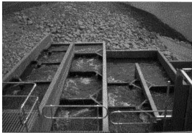
Below: A two cell vertical slot fishway
