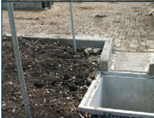
Effluent management from feed pads
