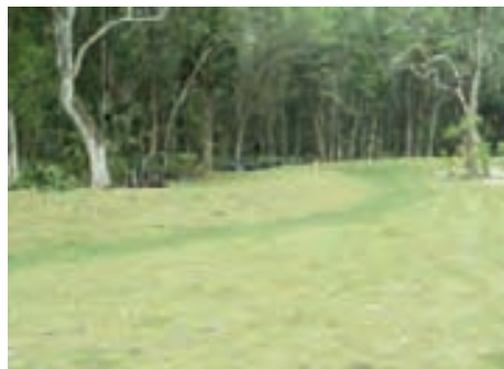
A broad curve is the most stable shape for a channel. Source: Grant Witheridge
