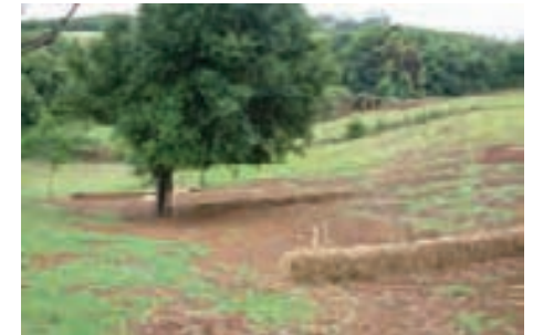
Hay bale check structures
