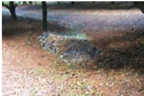
A small rock check structure
