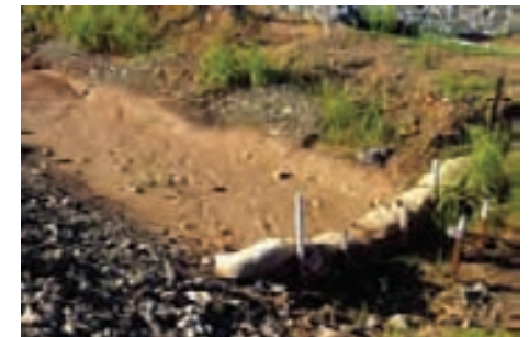
Check structure made from sandbags Source: Michael Frankcombe IECA
