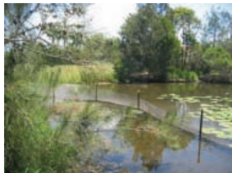
Install containment fences. Photo: Paul O'Connor
