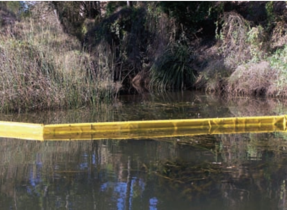
Install floating booms. Photo: Graham Prichard
