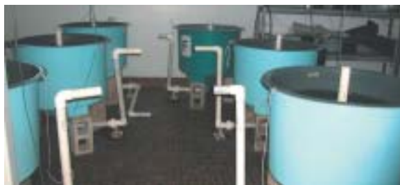
Fig. 6.7 Tanks (500L) used for incubation of eggs, holding fingerlings or quarantine; external standpipe controls water level and internal pipe screens the water.
