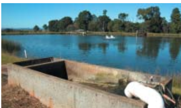
Fig. 6.3 Reservoir at Grafton Aquaculture Centre showing inlet, aerator and outlet tower.
