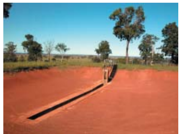
Fig. 4.5 Dry larval rearing pond showing internal harvest sump.
