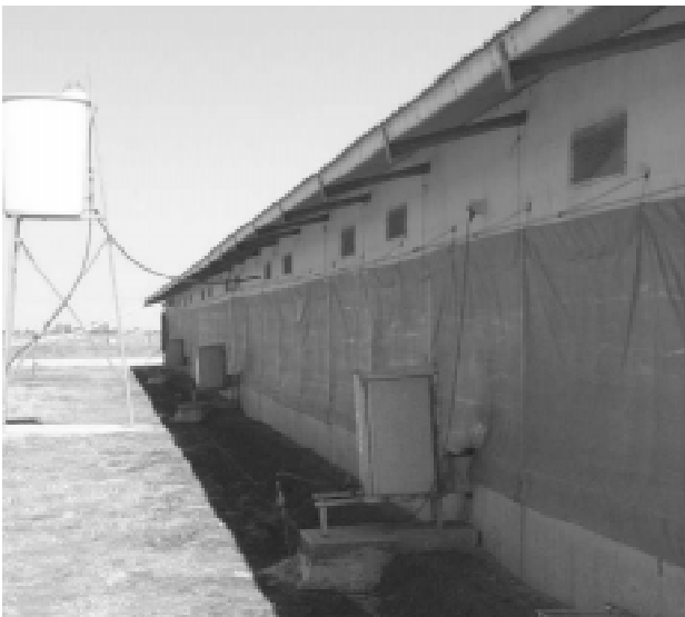
Heater units fitted to sheds are used to warm the shed for young birds.
