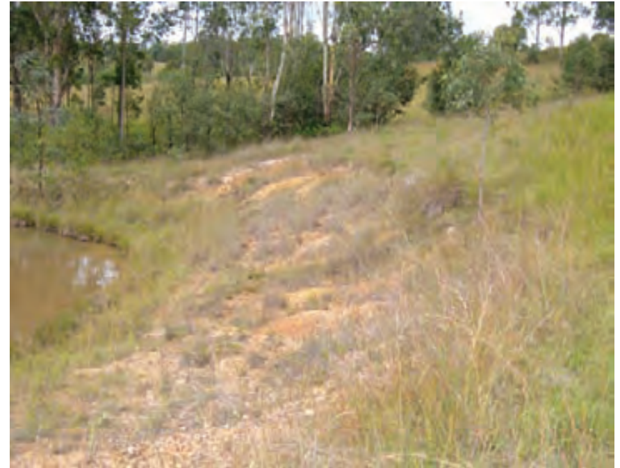
Exposed subsoil of the back batter is difficult to revegetate.
