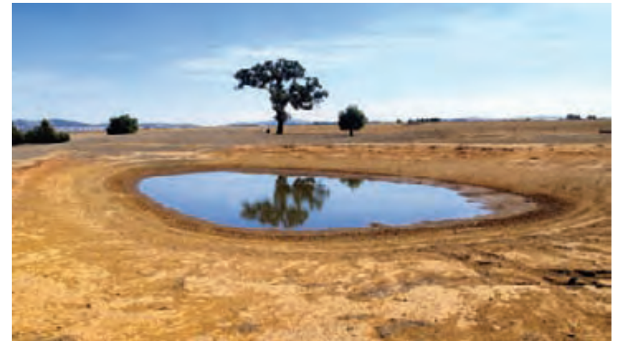
Excavated tank Source: Graham Johnson NSW DPI
