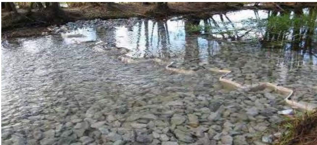
Corrosion-resistant vinyl sheet piling being used to retain groundwater
