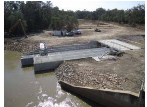
The vertical slot fishway at Marebone Weir. Photo: NSW DPI
