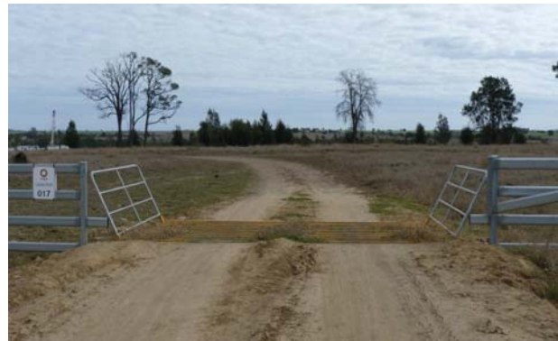
Figures 4 and 5: Access roads can be upgraded and cattle grids installed as part of an access agreement
