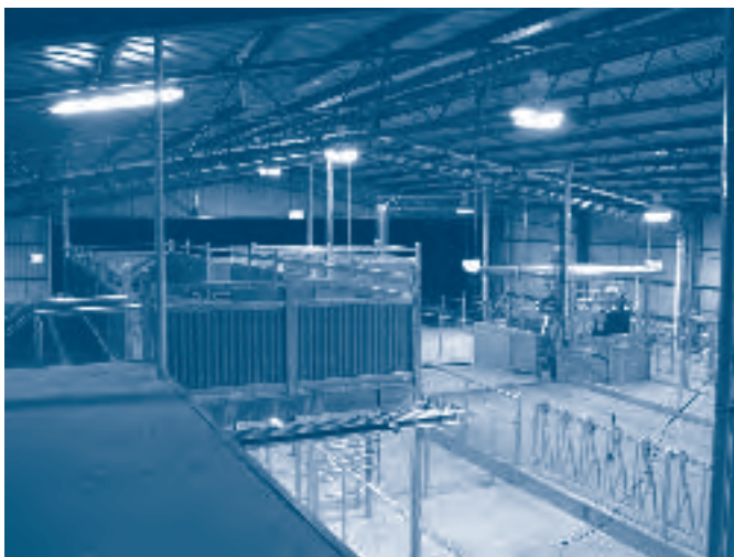
New automatic dairy constructed as part of the FutureDairy project at Elizabeth Macarthur Agricultural Institute, Camden.
