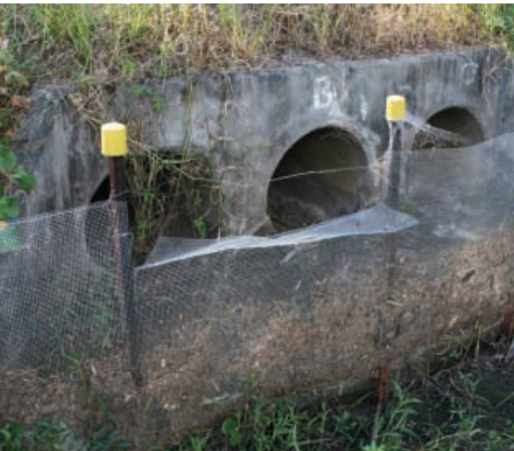
Fine mesh and star picket containment fence showing signs of wear and tear after 12 months' use. Photo: Elissa van Oosterhout
