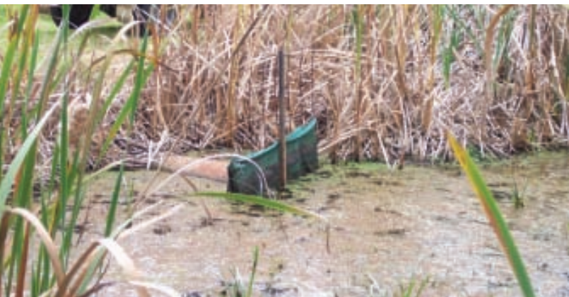
Shadecloth screen over culvert.
