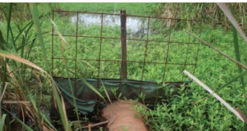
Screen made from reinforcement mesh and shadecloth.
