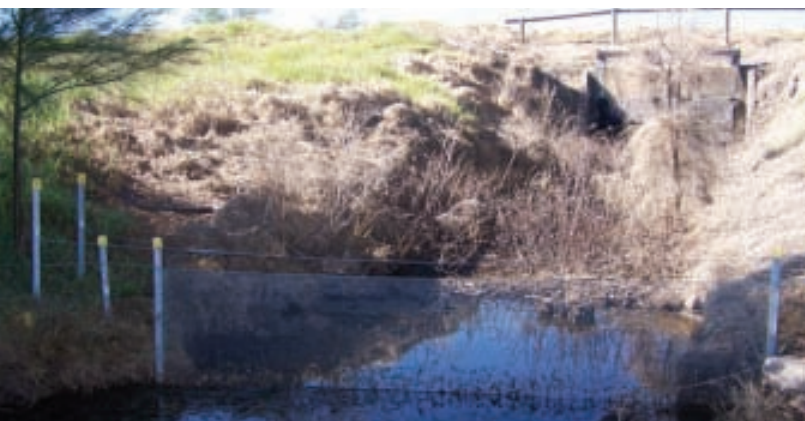
Fine mesh containment fence. Above photos: Graham Prichard
