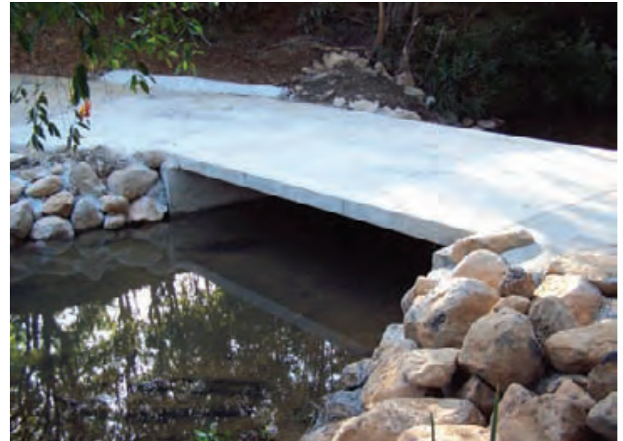
This modern box culvert causeway is more 'fish-friendly' than the older style.
