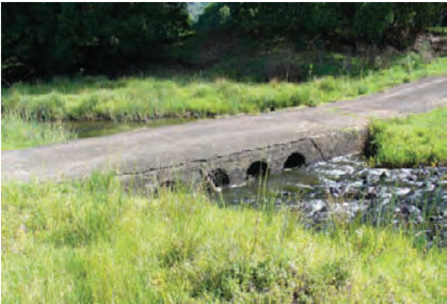
This older style culvert crossing is designed to function as a causeway in high flows.
