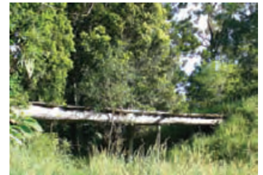
A timber bridge spans a deeply incised stream channel.
