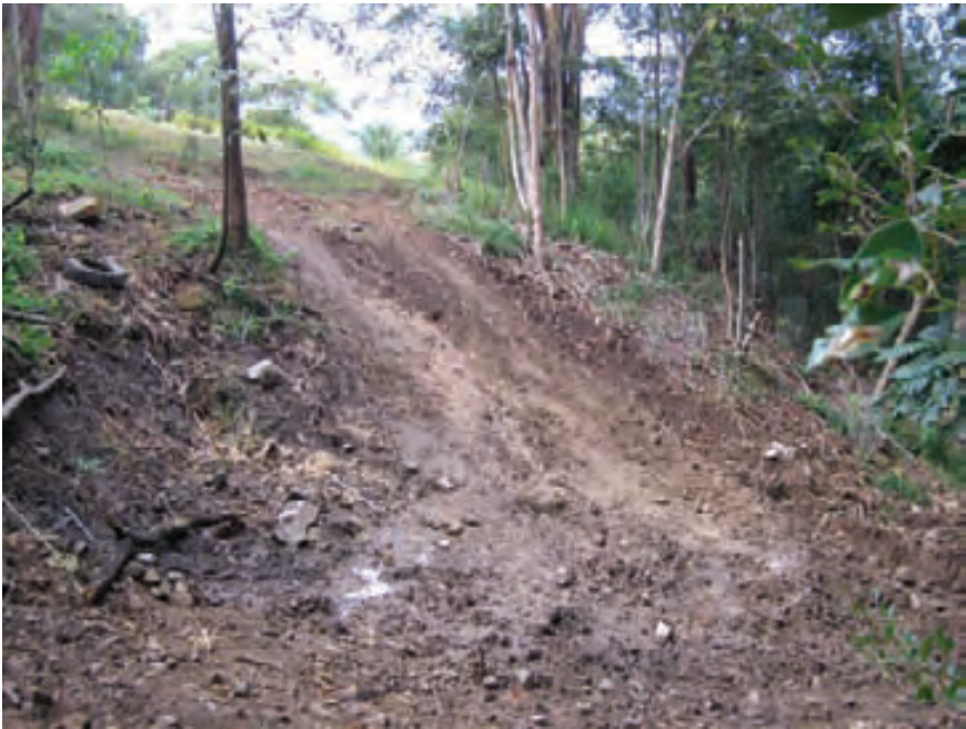
Lack of drainage and use in wet conditions have eroded this track.
