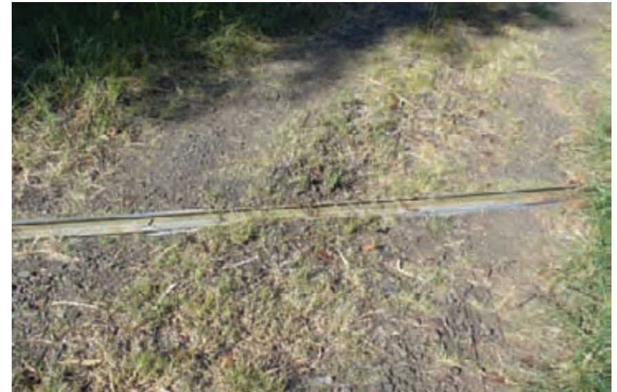
A recessed pipe set into a steep gravel track.
