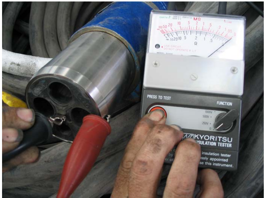
Figure 23: Earth continuity test from phase barrier to nose-cone for a typical 150 Amp restrained plug
