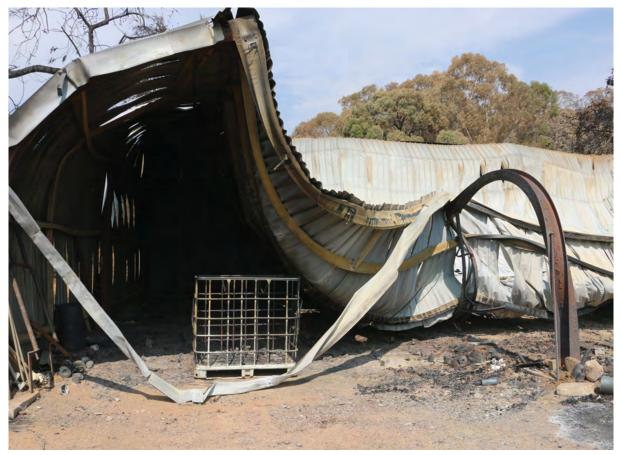
Figure 27. A harvest bin storage shed generated enough heat to soften and bend steel beams. Photo taken 10 January 2020, 6 days post-fire.
