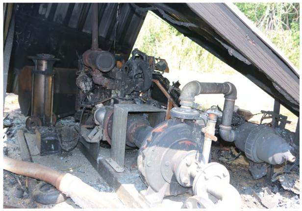
Figure 28. Damage to irrigation pumps hampered efforts to re-establish irrigation to the orchard following the fires. Photo taken 10 January 2020, 6 days post-fire.
