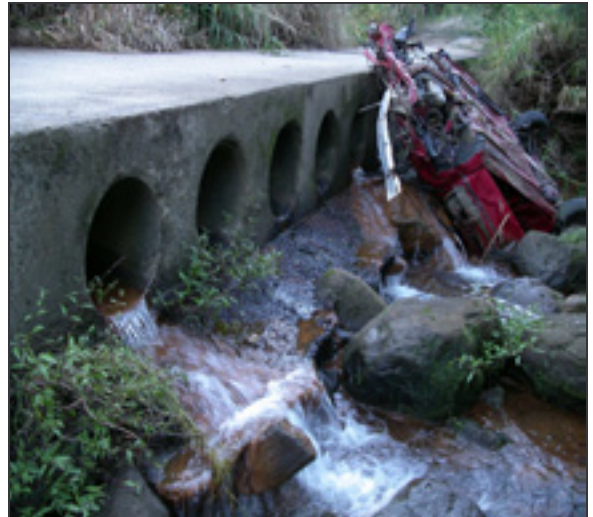
Photo 2. Pipe culvert with high invert (headloss) (Fitzgeralds Ck, Lower Hawkesbury-Nepean subregion)
