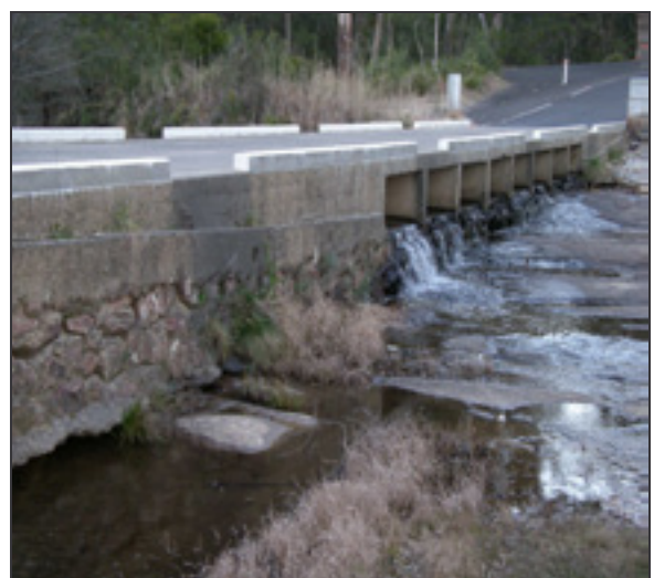
Photo 4. Box culvert with high invert (headloss), and low flow depth (Megalong Ck, Upper Hawkesbury-Nepean subregion)
