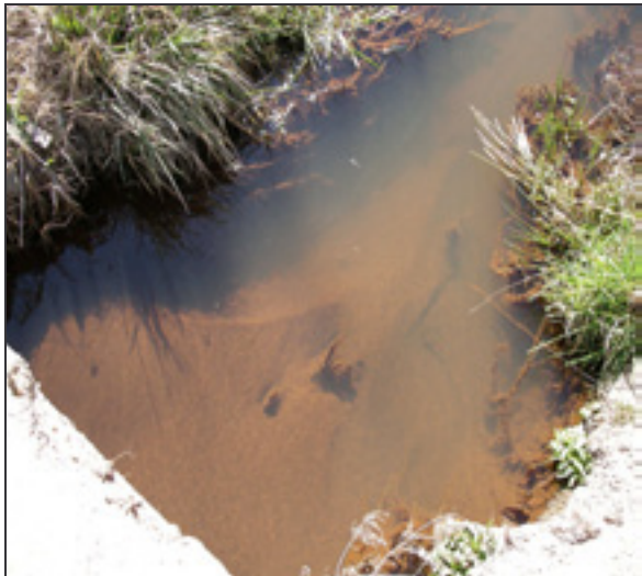
Photo 3. Box culvert on unsealed road producing sediment inputs (Cullenbong Ck, Upper Hawkesbury-Nepean subregion)
