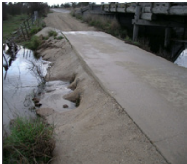
Photo 7. Redundant causeway with inadequate pipes adjacent working bridge (Mulwaree R, Upper Hawkesbury-Nepean subregion)
