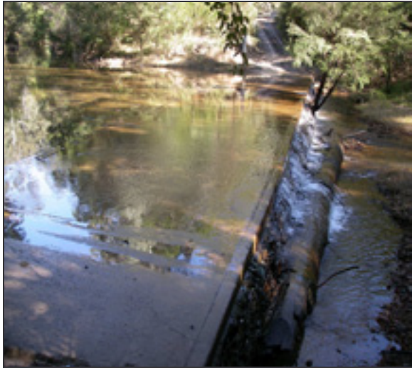
Photo 1. Causeway with high invert (headloss) and shallow water depth (Wheeny Ck, Lower Hawkesbury-Nepean subregion)
