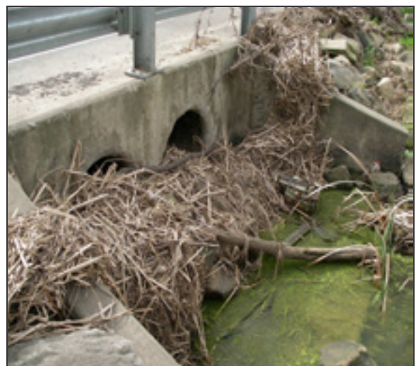
Photo 8. Pipe culvert with excessive debris (Kemps Ck, Lower Hawkesbury-Nepean subregion)
