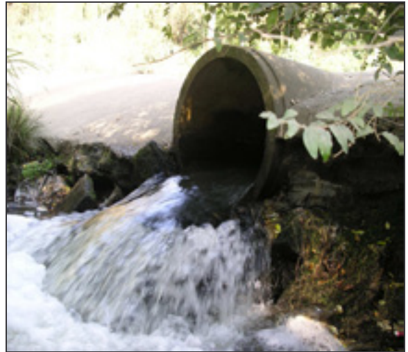
Photo 6. Pipe culvert with high invert (headloss) and increased water velocities (Cattai Ck, Lower Hawkesbury-Nepean subregion)
