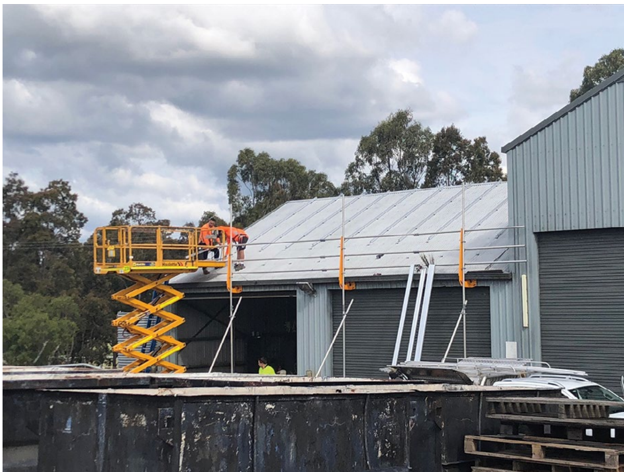
Figure 15. Lift and edge protection in use during solar installation.
