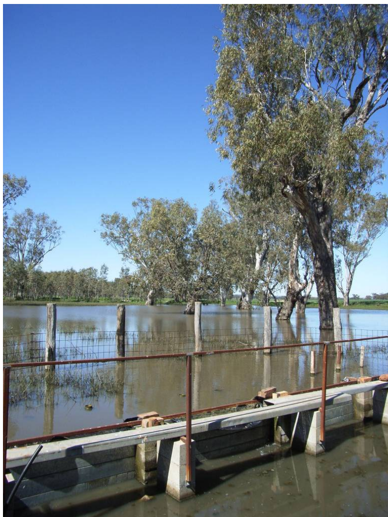
Image 27: Drained in the 1950s, the flow of water in and out of the wetland at Dappo is now controlled by a levee bank and this small weir constructed in 1999.
