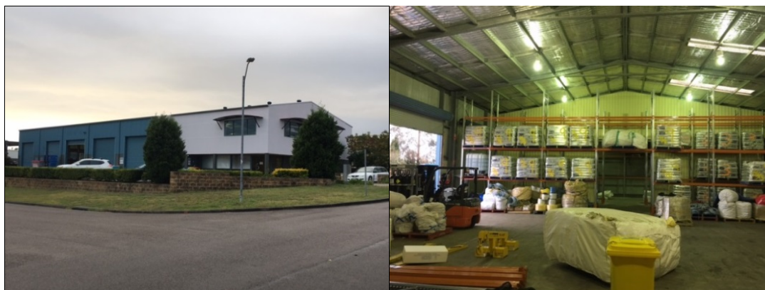
Huon's new land based facility at Taylors Beach
