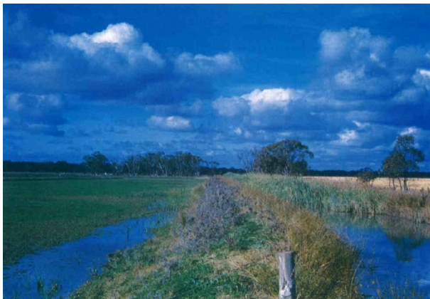
Figure 27. Irrigation channel and shallow drainage area.
