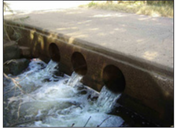
Photo 2. Pipe culvert with high invert (headloss) (Black Ck, Hunter subregion)
