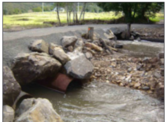
Photo 10. Pipe culvert with high water velocities (Crawford R, Hunter subregion)
