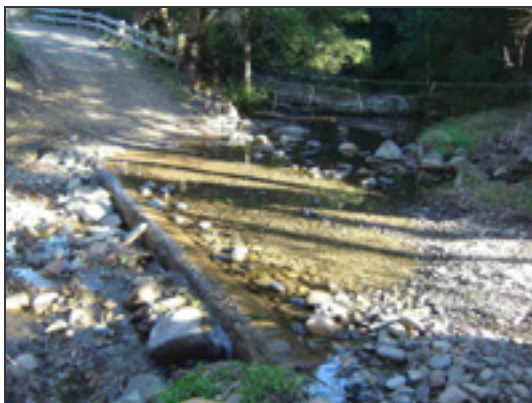
Photo 9. Ford with high invert (headloss) (Berrico Ck, Lower North Coast subregion)
