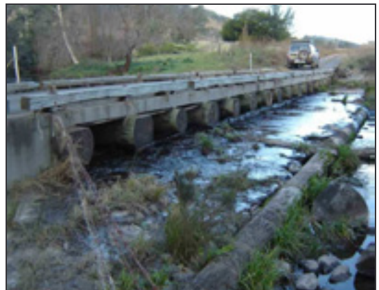
Photo 8. Combination structure (causeway used as low bridge base), high invert (headloss) and shallow water depth (Belbora Ck, Lower North Coast subregion)
