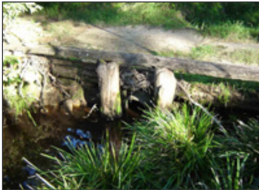
Photo 3. Piped crossing with inadequate sized pipes, and high invert (headloss) (Morans Ck, Central Coast subregion)
