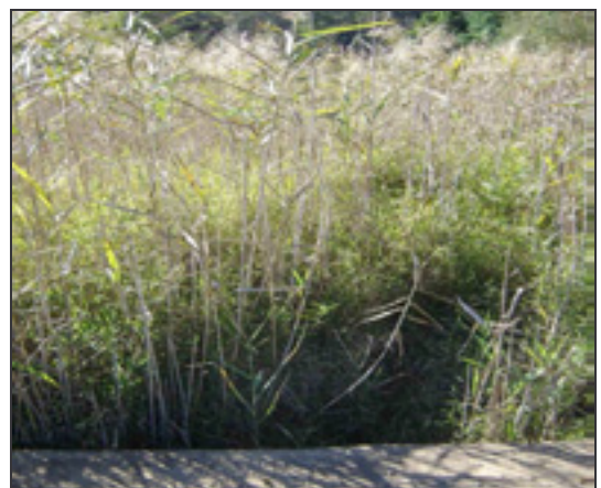
Photo 12. Pipe culvert with excessive reed growth (Wollumbi Ck, Hunter subregion)
