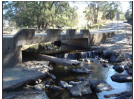
Photo 4. Bridge with scouring on downstream side creating headloss (Berrico Ck, Lower North Coast subregion)
