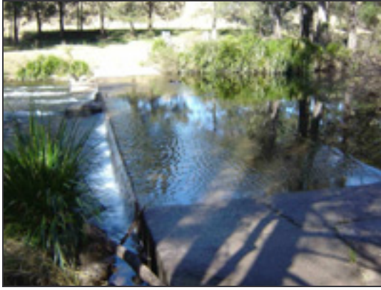
Photo 1. Causeway with high invert (headloss) and shallow water depth (Manning River, Lower North Coast subregion)
