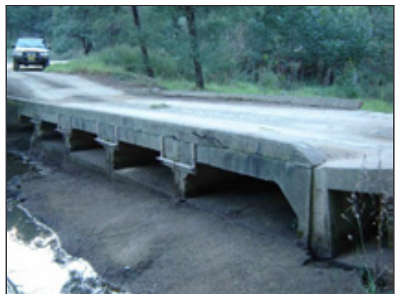
Photo 6. Low box culvert with steep apron (Wollombi Ck, Hunter subregion)
