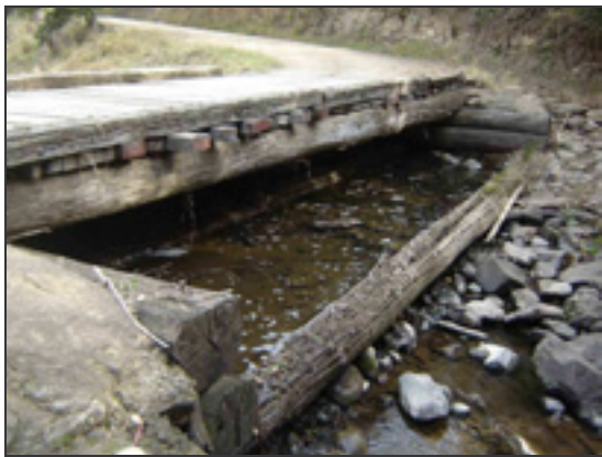
Photo 7. Combination structure (causeway used as low bridge base), high invert (headloss) and shallow water depth (Firefly Ck, Lower North Coast subregion)
