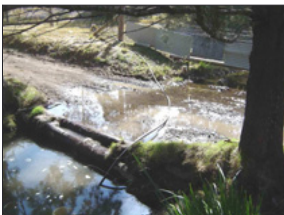
Photo 11. Ford crossing with high invert (headloss) and increased sediment loading (Bullen Bullen Ck, Lower North Coast subregion)
