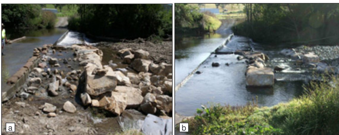
Figure 5. Faulkland Road Crossing modified partial width rock ramp fishway (a) during construction, (b) completed work.
