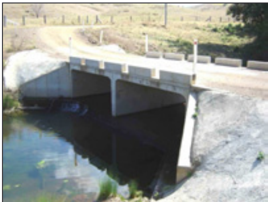
Photo 5. Box culvert with high invert (headloss) and shallow water depth (Kerriki Ck, Lower North Coast subregion)
