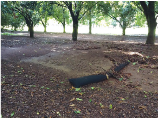
Check structures that fill with sediment must be cleaned out for continued benefit.
