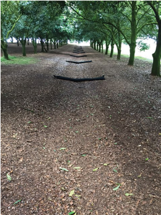
Temporary check structures made from geotextile fabric, filled with blue metal, slow water on a bare inter-row drain. These are removed for harvest.
