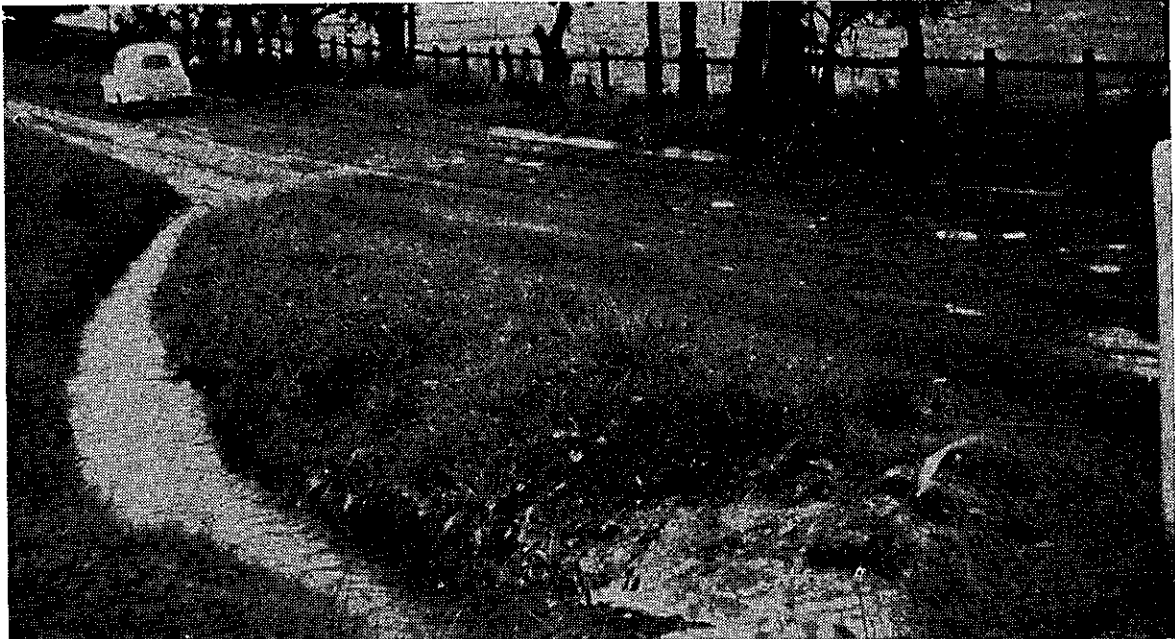
Roads are often good sources of water for filling dams. The illustration shows a table-drain discharging water into a culvert which feeds a roadside dam at Badgery's Creek.
