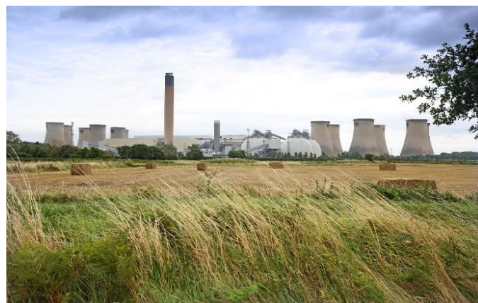
Figure 3: Drax power station in the UK.
