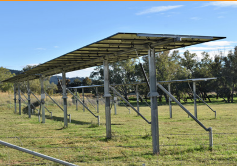
Left: Agrivoltaics – allow the simultaneous use of land for both solar PV power generation and agriculture. In this case the PV panels have been raised and the frames structurally reinforced to allow grazing of cattle in the same paddock as the panels.
