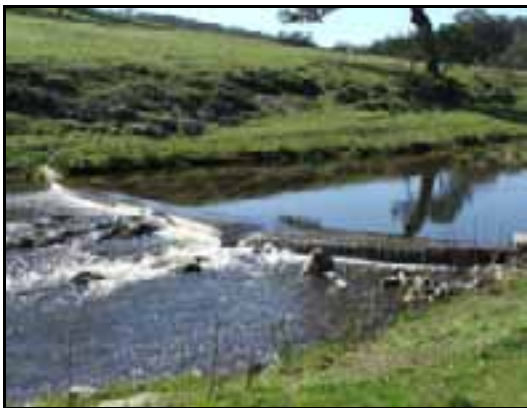
Plate 33: Swamp Oak Creek water gauge (WGS7)
