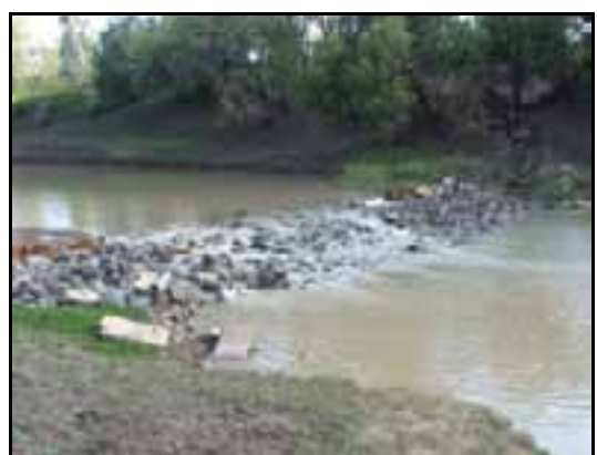
Plate 12: Walgett Weir (419/970000/B0068)
