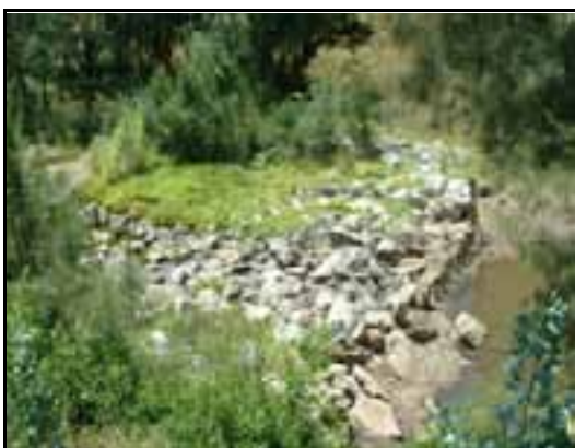
Plate 5: Bed control structure, Cockburn River, Tamworth LGA (Code: BCS8).
