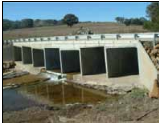
Plate 15: Mayvale Road Culvert (UMA76)
