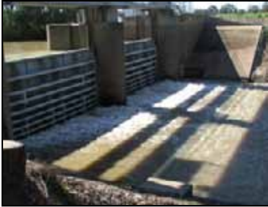
Plate 1: Gunidgera Weir, Namoi River, Narrabri LGA (Code: 419/970000/B0104).
