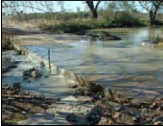
Plate 23: Pian Creek Causeway (LPC13)
