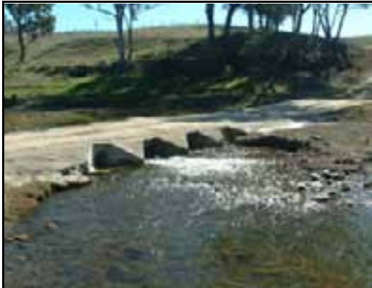
Plate 29: "Plumthorpe" Culvert (UMA73)
