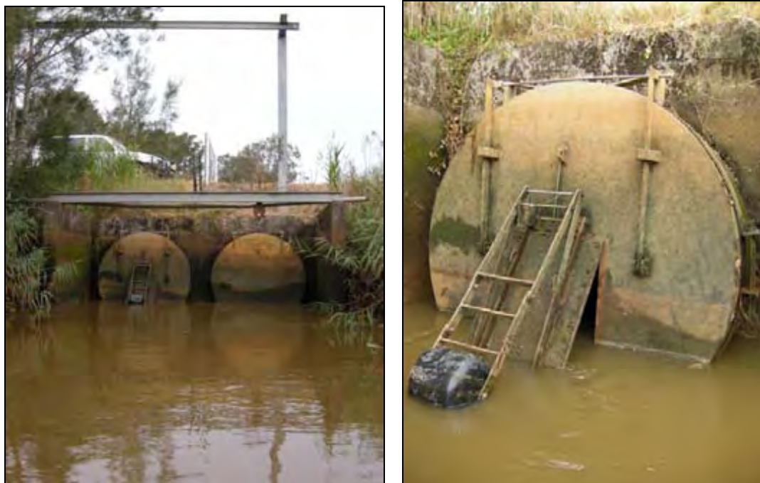
Figures 4 & 5 Auto-tidal floodgate on Windeyers Creek (Raymond Terrace) similar to the recommended management recommendation for Tilligerry Creek floodgates.
