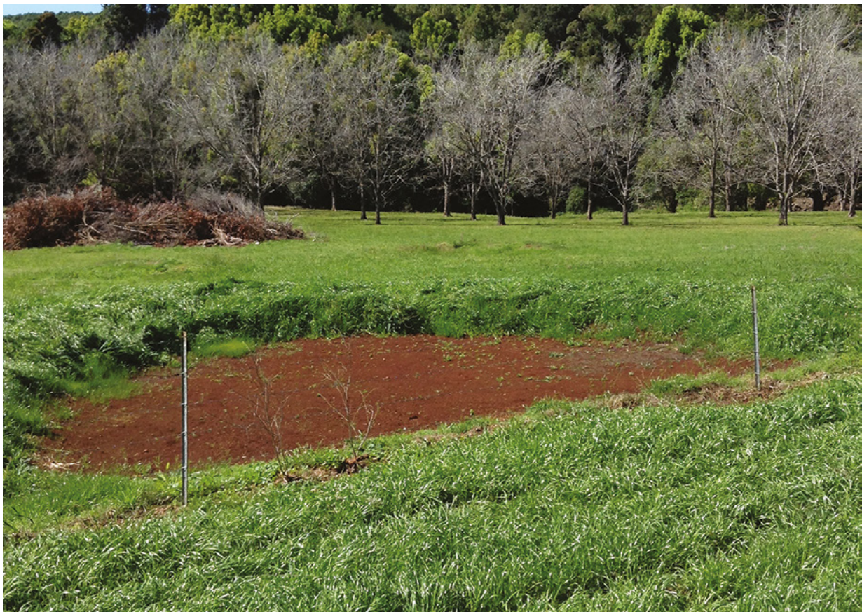
Figure 41. A sediment pond catches soil so it does not leave the property.
