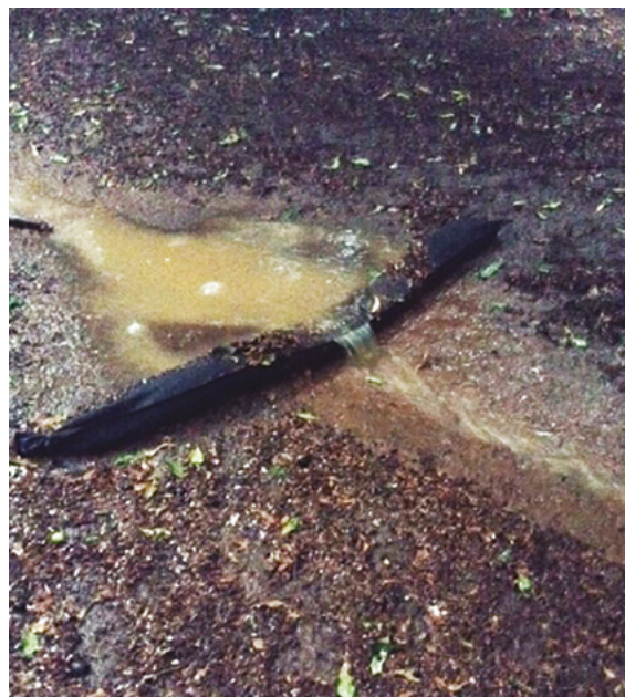
Figure 39. An erosion control 'sock' used in a bare inter-row drain as an interim measure.
