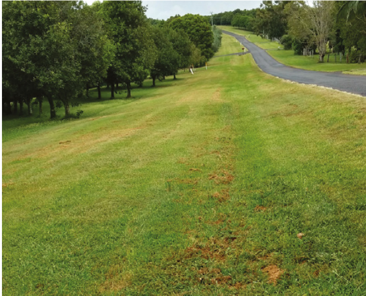
Figure 10. Water from the road is directed around the tree block.
