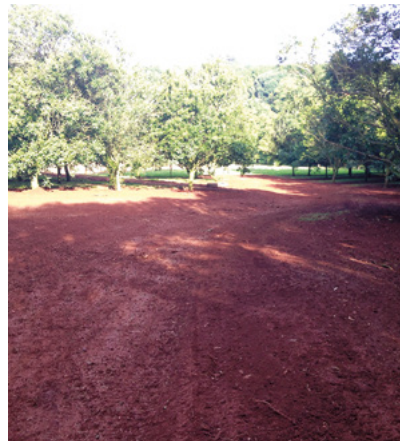
Figure 19. Earthworks shape the watercourse.
