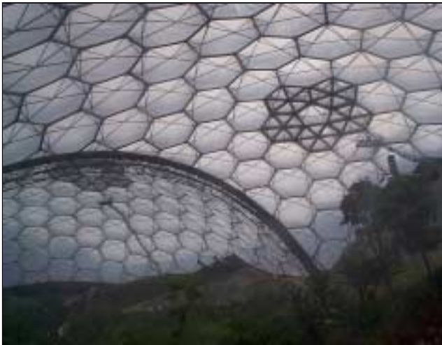
The massive biomes are made up of hundreds of triple layer foil panels. The triangular panels are air vents.
