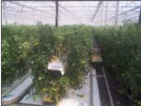
A media based system is raised off the ground to assist airflow and management.
