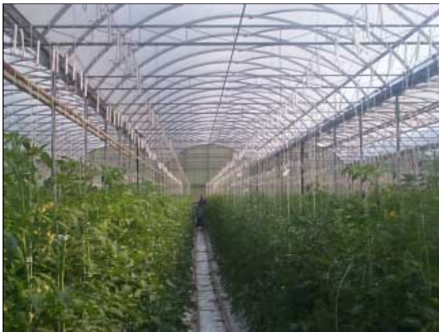
Curved glass is a new development by a Canadian manufacturer, which offers the improved light transmission of both glass and a curved roof design.
