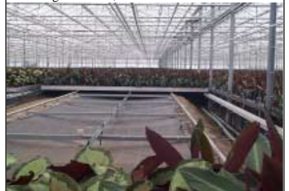
Below: Water storage reservoirs are constructed in the greenhouse, beneath the mobile benches.
