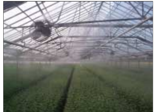
High pressure fogging systems assist cooling and relative humidity management without wetting the crop..
