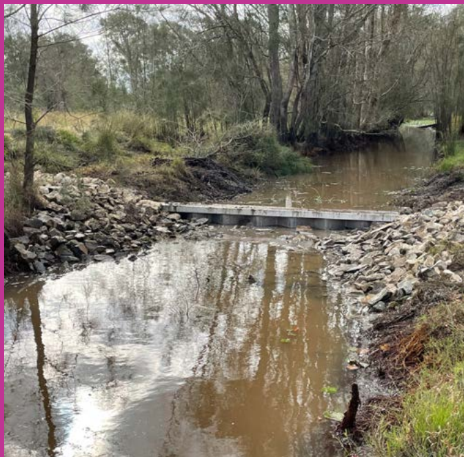
📷 Newly installed weir in Clybucca across the East Drain
