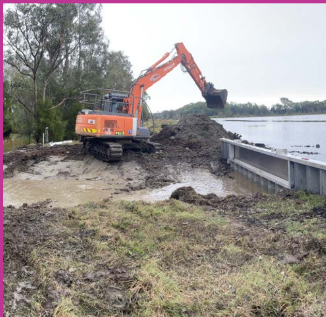
📷 Weir being installed in Clybucca at the Southern Scald
