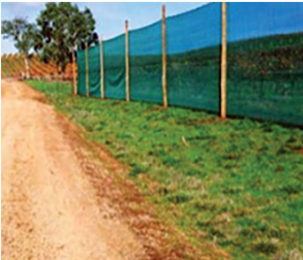
Figure 12. An artificial barrier made of shade cloth with 50% porosity. Photo: Andrew Hewitt.
