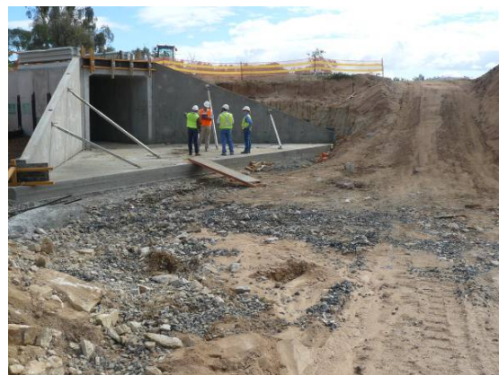
New boxed culvert tunnel under construction
