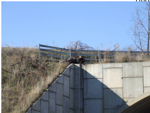
Safety barrier positioned above tunnel entrance
