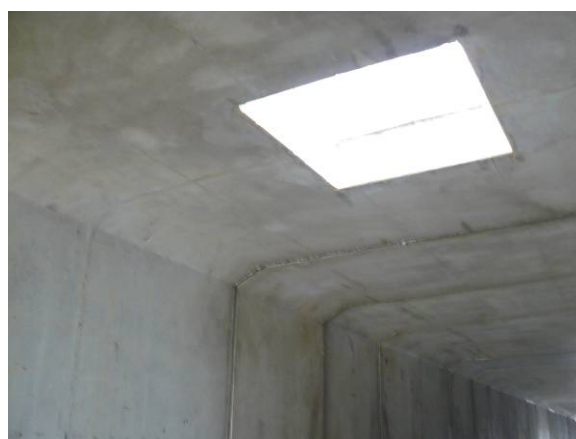
Skylight producing direct light – this light should be diffused to stop animals balking at shadows
