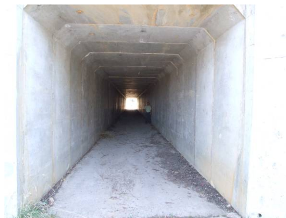
Stockman standing fifteen metres from tunnel entrance
