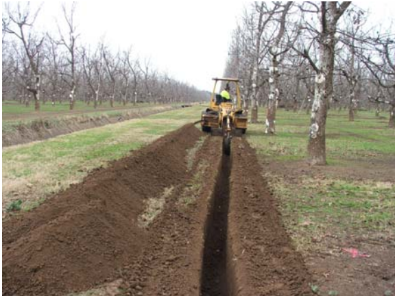
Establishing the trench for the main line. Image: S Bray
