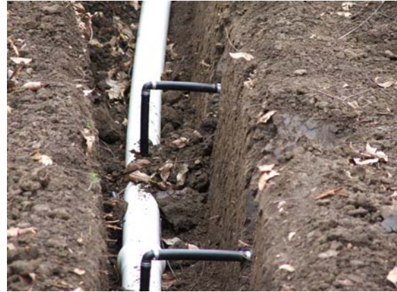
The two lines of dripper tape coming off the main line. Image: S Bray
