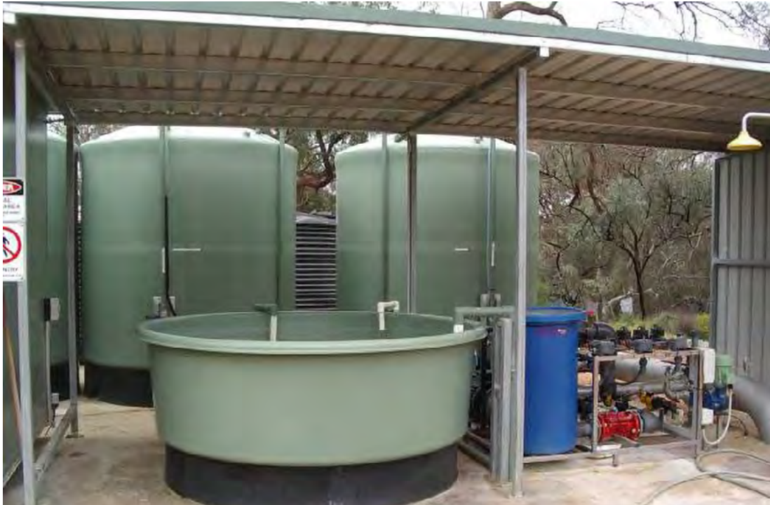
Figure 2. Fully automated twin multi-tank fertigation system.
