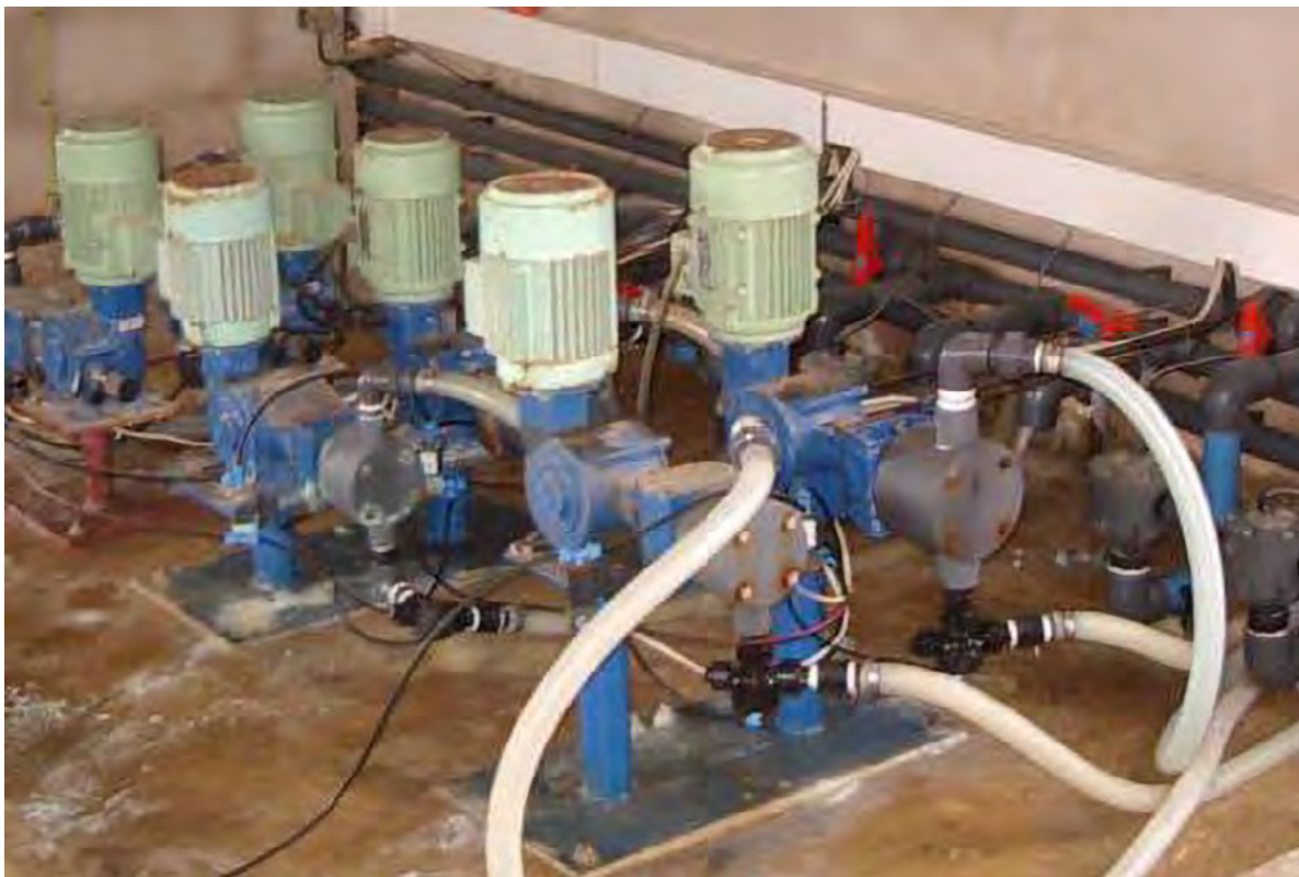
Figure 6. A set of six piston pumps used to run a multi-tank injection system.
