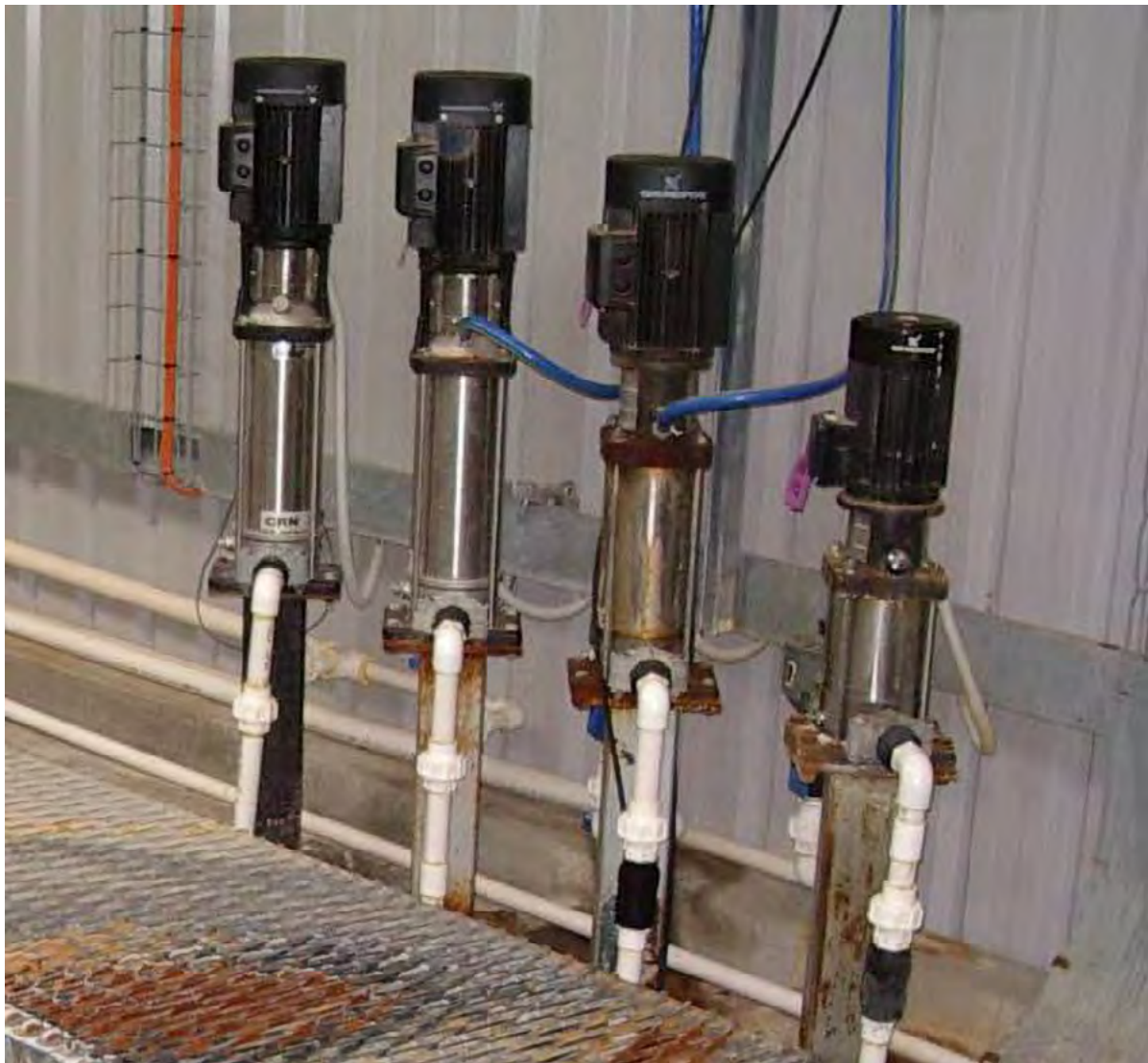
Figure 7. A series of multi-stage centrifugal pumps used to proportionally inject in a fully automated fertigation system.
